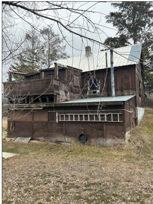
View from the West side of the property
