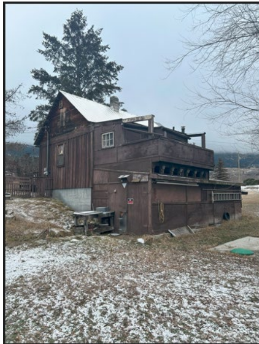
North west view of the structure
