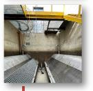
Vernon Creek Intake Screens Installation - Self cleaning screens installed for safer and more efficient operations
