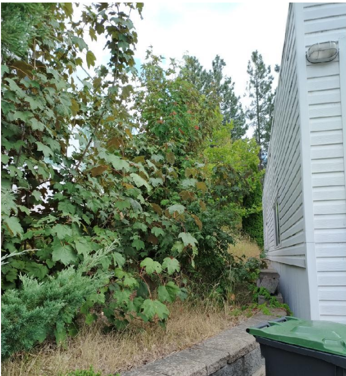
East side of structure to be replaced, flashy grass fuels along this side.
