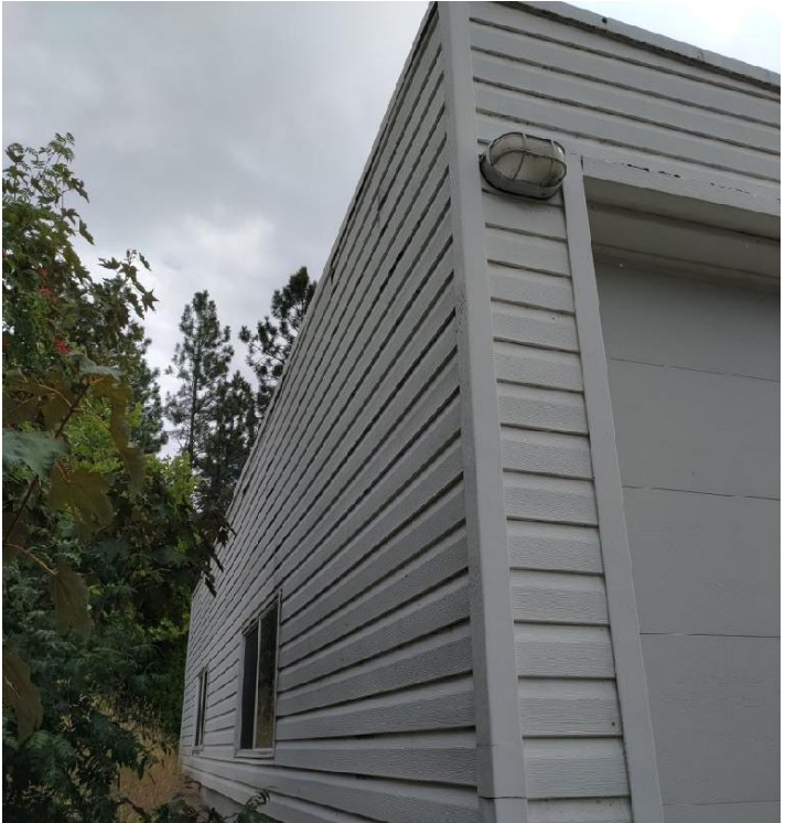
East side of existing structure to be replaced.
