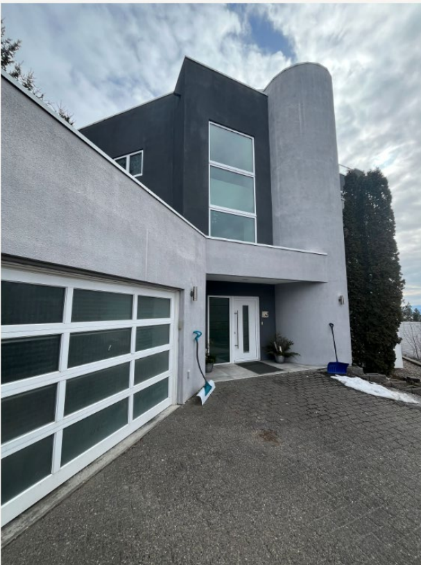
Front view of the existing structure from North
