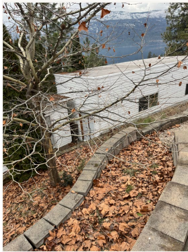
View from South (Garage)
