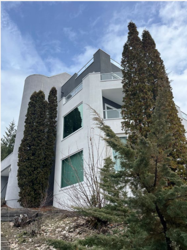
West side view of existing structure
