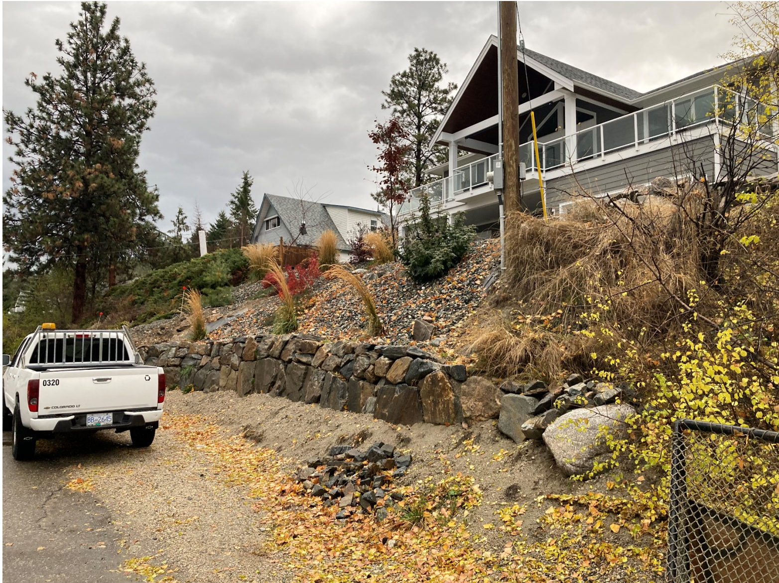
Figure 4: 17073 Coral Beach Road; Stone retaining wall displayed is at 50% completion.
