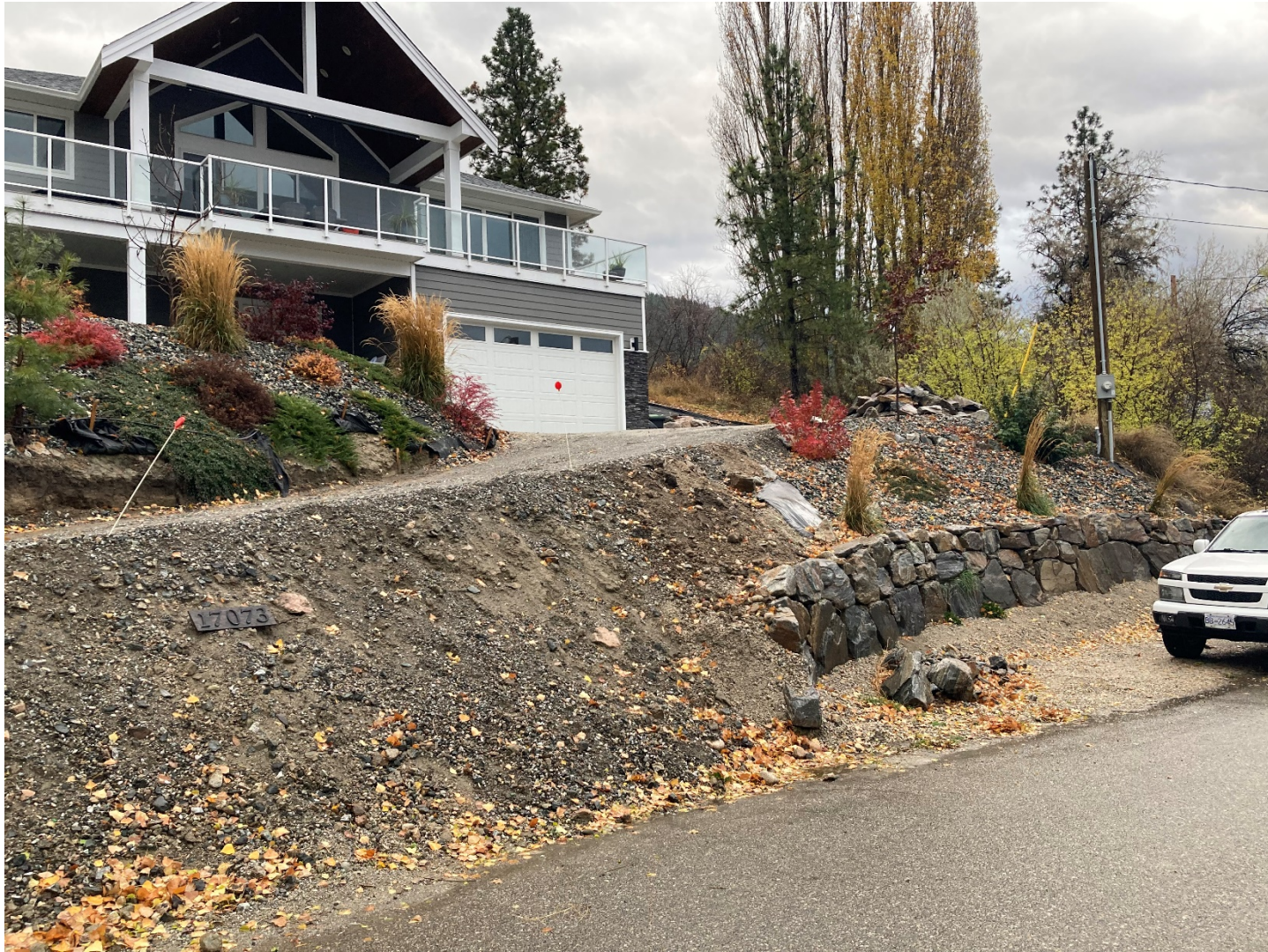
Figure 3: 17073 Coral Beach Road; Stone retaining wall displayed is at 50% completion.
