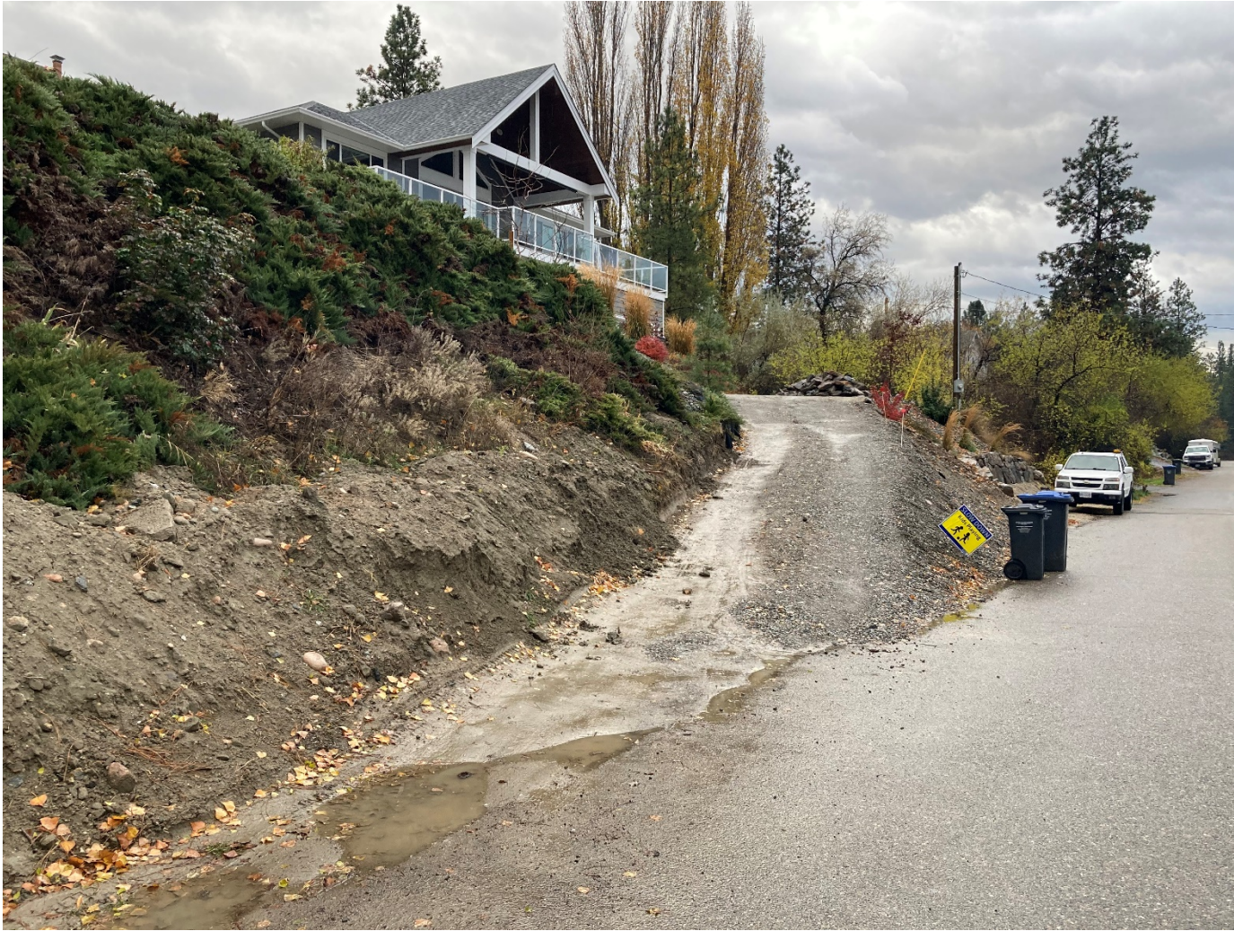
Figure 2: 17073 Coral Beach Road driveway (looking south). Existing driveway toe of slope extends to edge of pavement.
