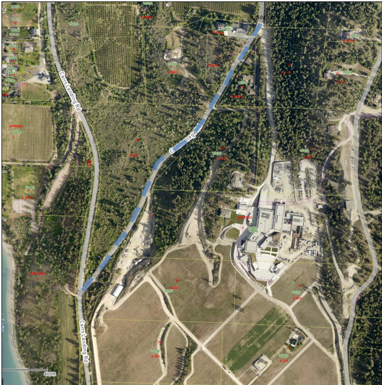
Figure 2: ORFV required road/mobility improvements on a portion of Commonage Road
