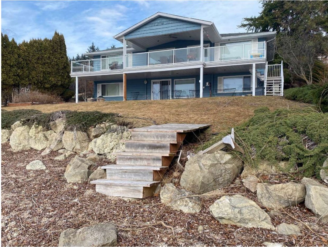
Photo 1: Looking towards the subject property and the existing single-family dwelling (March 5, 2021).
