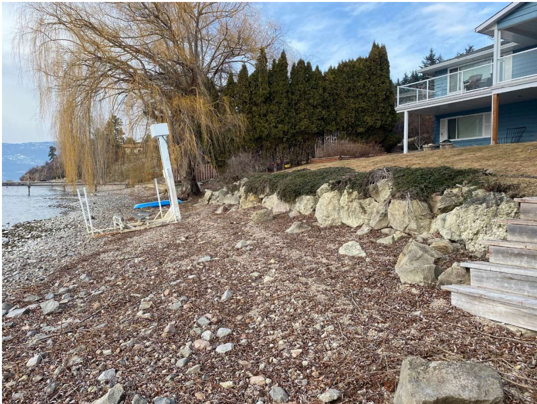
Photo 4: Looking northwest along the foreshore towards the boat lift remaining from the previous moorage, rock retaining wall, and riparian condition (March 5, 2021).
