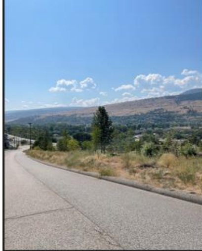
Photo 4: Robinson Road Slope
