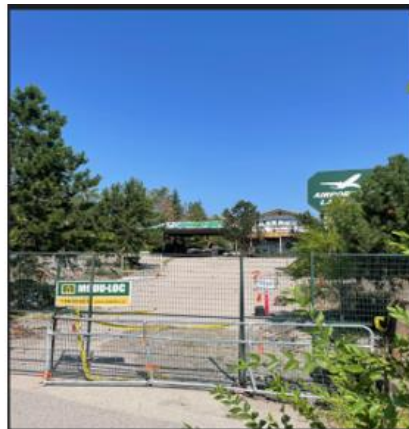
Photo 2 - Site entrance - Petrie Road
