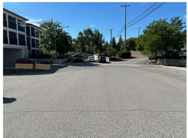
Photo 7: Powley Court – South
