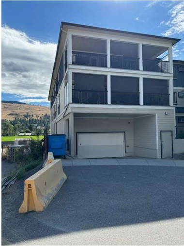
Photo 1: Adjacent property to South
