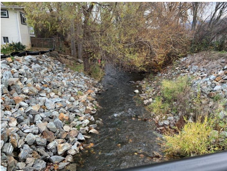
Reimche Road Downstream
