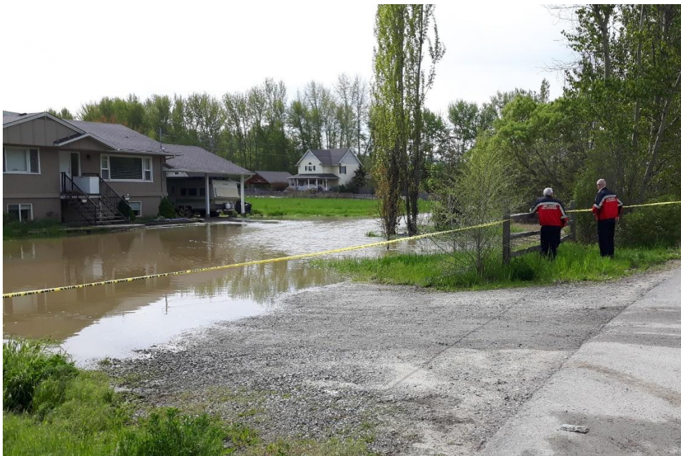
Figure 4.4. Flooded property along Middle Vernon Creek
