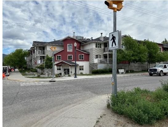
Photo 4: Adjacent multi unit residential buildings looking north
