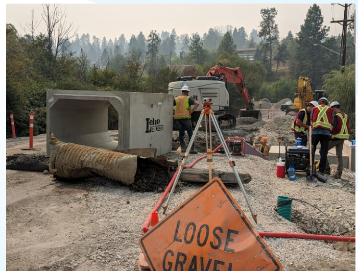
Installation of a new concrete box culvert to replace aged pipe culvert on the west end of Woodsdale Road.
