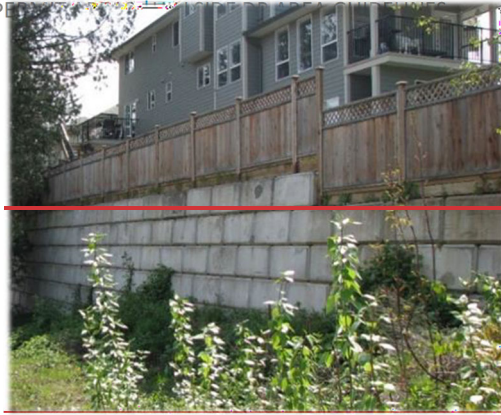
Example of Large concrete lock block that is not considered to be a context-sensitive retaining material and, if used, it should be masked or screened
