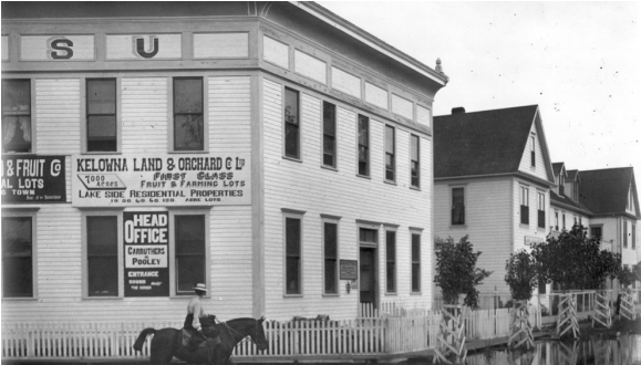
Bernard Avenue at Abbott Street
