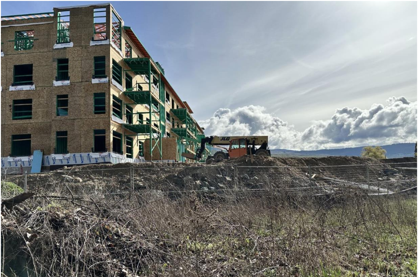
SITE PHOTO 2: LOOKING SOUTH
