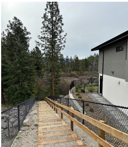
Photo 1: Walkway to public open space
