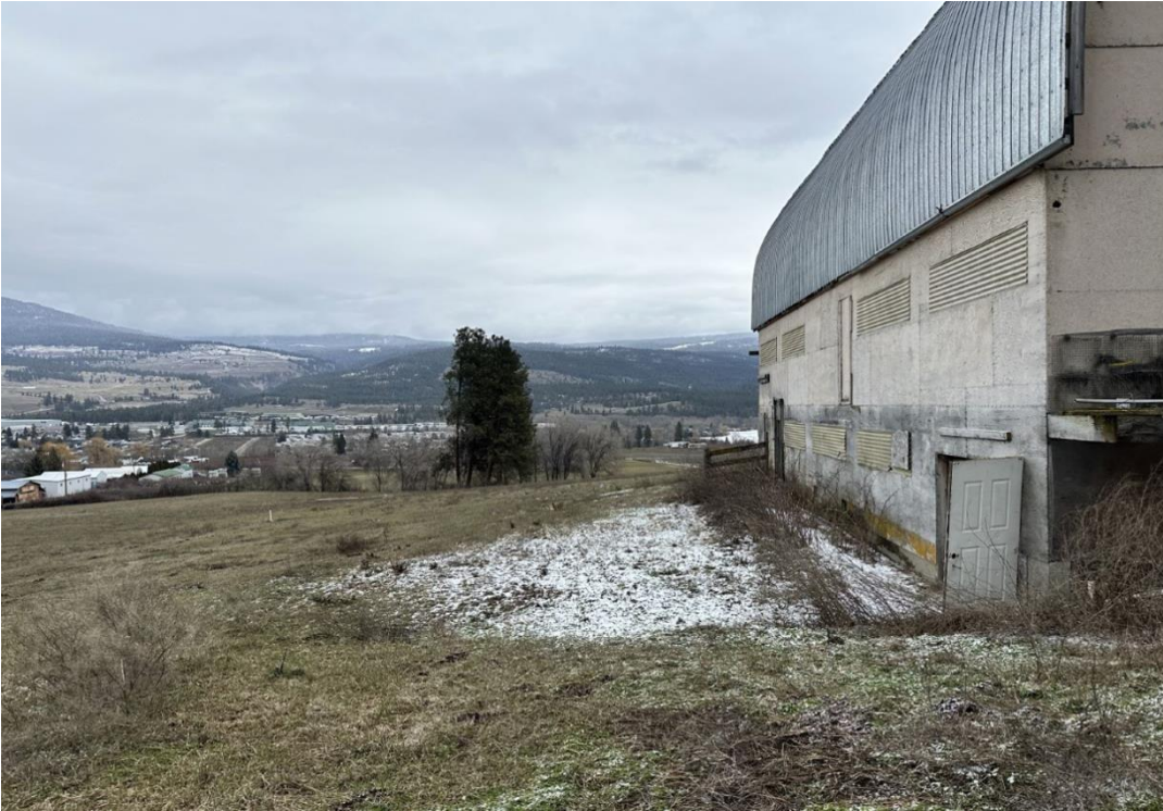
FIGURE 2: SITE PHOTO LOOKING EAST FROM THE NORTH SIDE OF THE BARN
