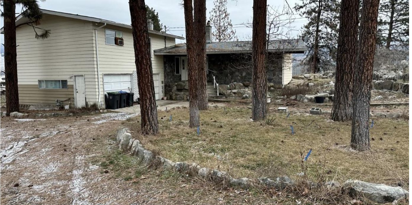
FIGURE 3: SITE PHOTO LOOKING EAST AT THE HOUSE
