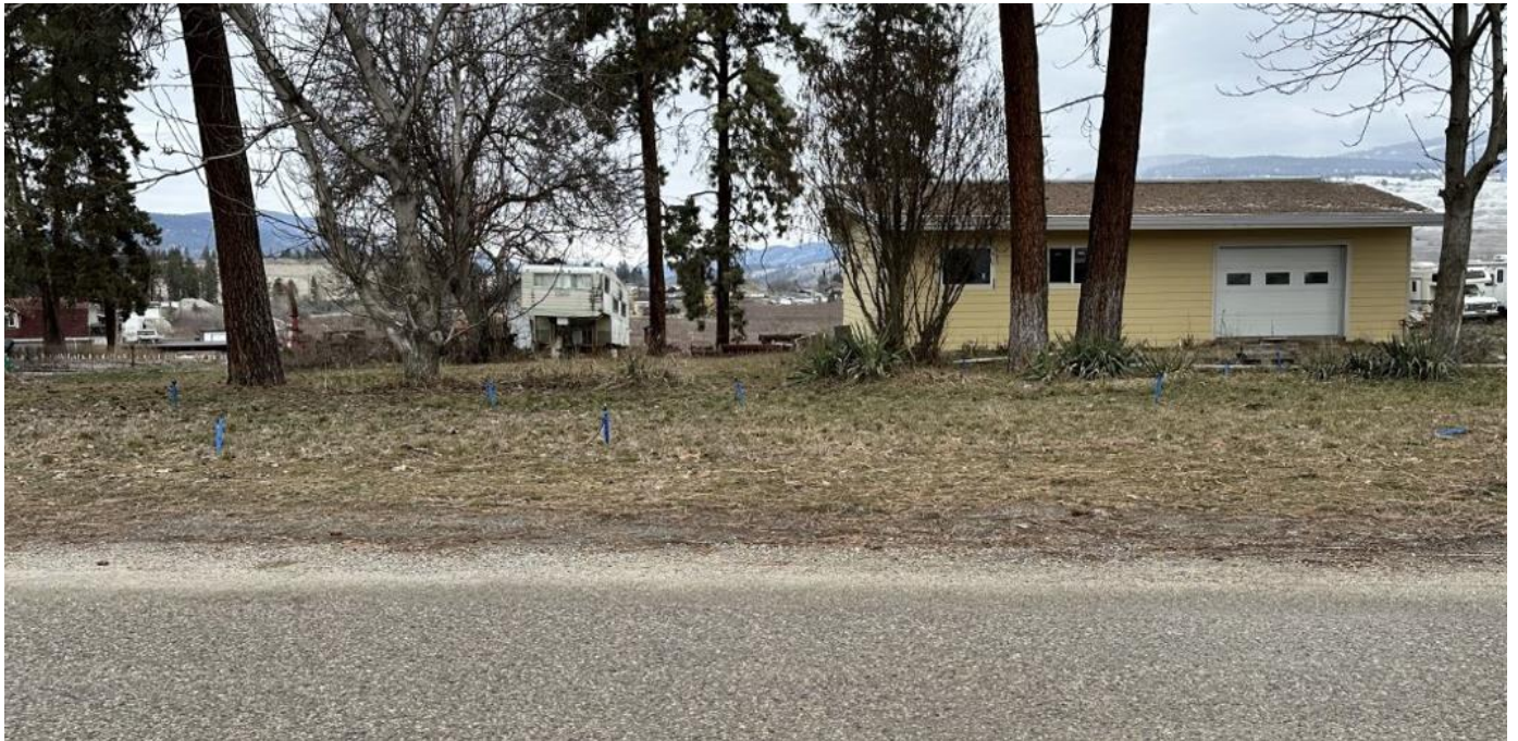
FIGURE 5: SITE PHOTO LOOKING NORTH FROM THE EAST SIDE OF THE HOUSE
