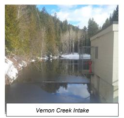
At the headworks of the Beaver Lake water source is the Vernon Creek intake. Before water enters the system, it passes through debris screens that are currently cleaned manually. Cleaning of the screens can be labour intensive, especially during freshet when turbidity increases. Screen blockages increase risks of water service interruptions and damage to the pipe systems that feed into the Eldorado Raw Water Reservoir.
