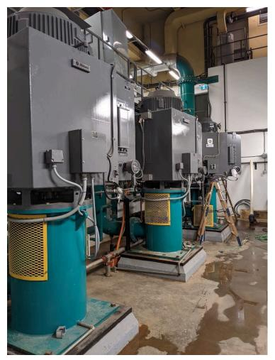
The Okanagan Lake Pumphouse is equipped with three 750HP high-capacity pumps, which are responsible for supplying water to the Okanagan Lake distribution system. This facility is the largest supplier of domestic water within our community, thus making it critical to ensure continued smooth operation.
