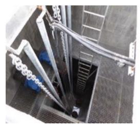
Image above shows a lift station with a platform to work from
