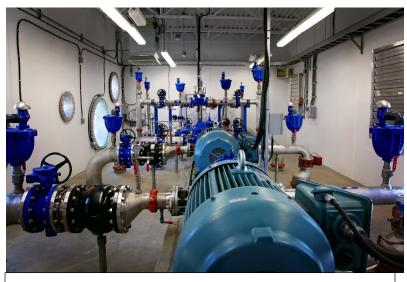
Picture of the Glenmore Booster Station. This facility pumps Okanagan Lake water into the Beaver Lake Distribution System
