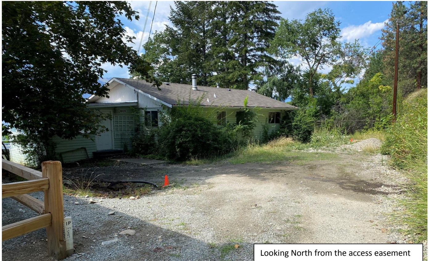
SITE PHOTO 1: NORTH VIEW FROM AN ACCESS EASEMENT
