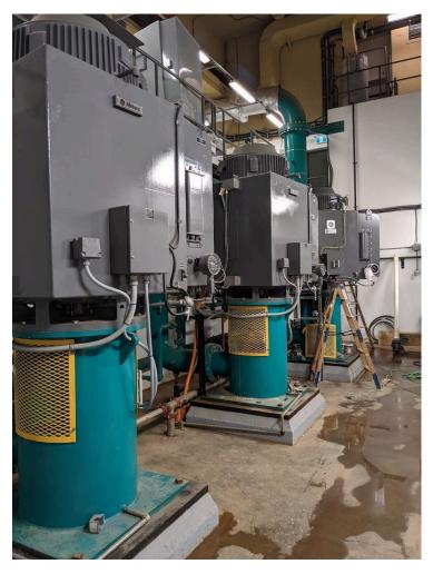
The Okanagan Lake Pumphouse is equipped with three 750HP high-capacity pumps, which are responsible for supplying water to the Okanagan Lake drinking water source. Two of the motors were purchased and installed in 2008, and the third in 2021.
