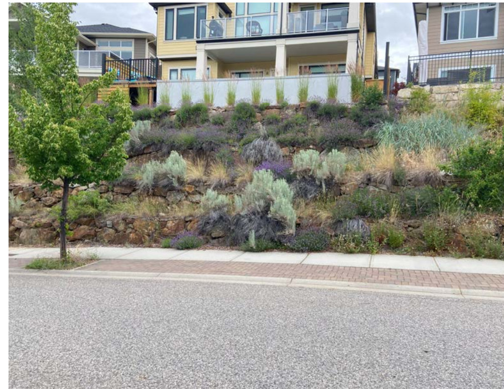
3 WALL SCREENING EXAMPLE PHOTO R02
